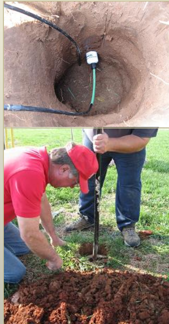
Soil Probe Installation
